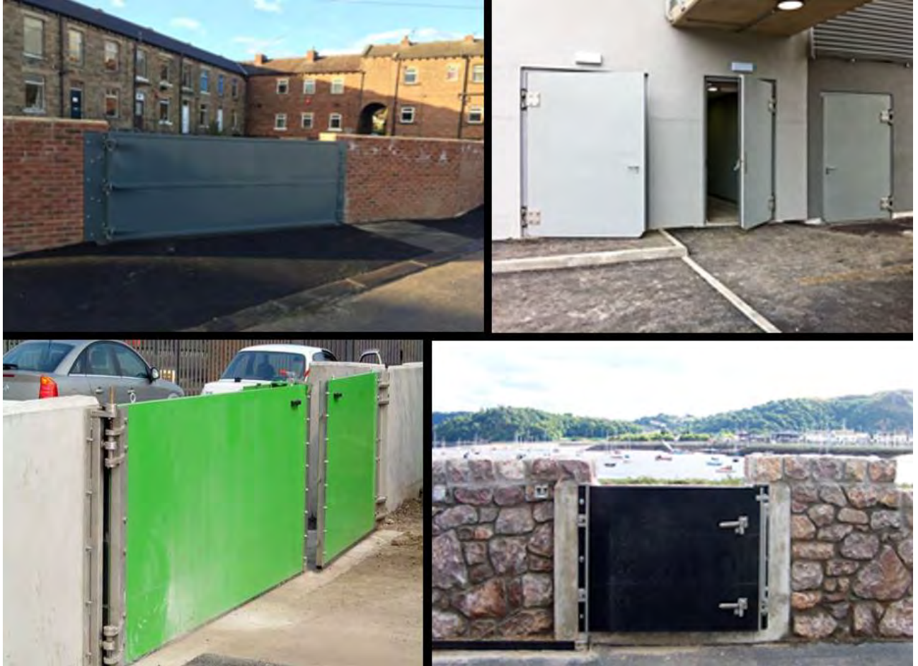
Figure 7-2 Typical Examples of Swinging Flood Doors
