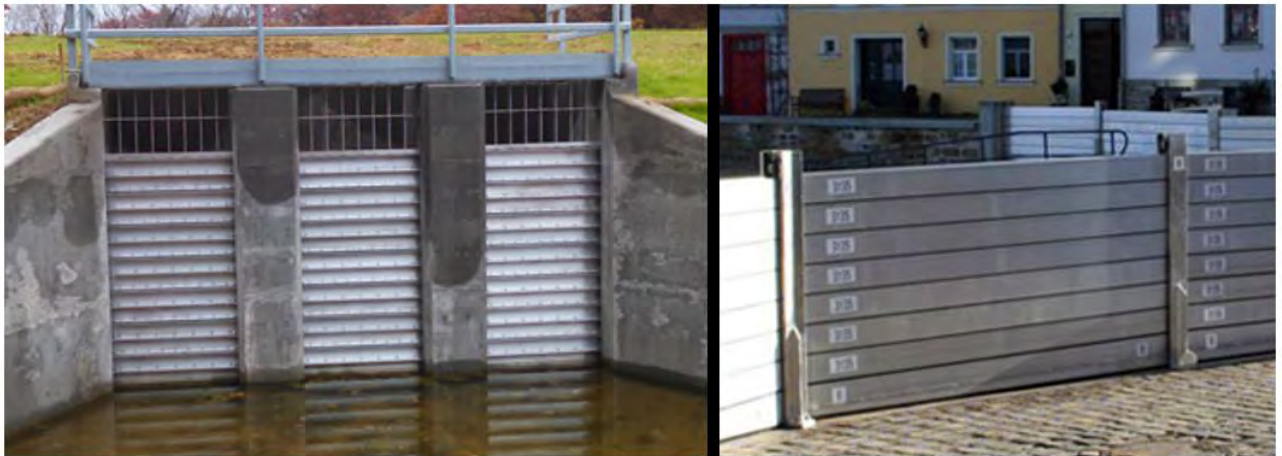
Figure 7-1 Typical Floodwall Stop Log Examples
