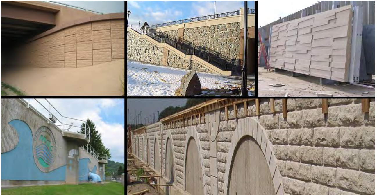
Figure 7-4 Typical Examples of Floodwall Cast Patterns
