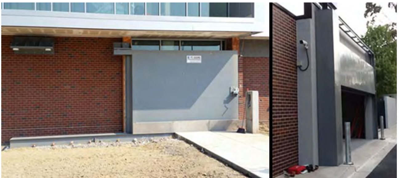
Figure 7-3 Typical Examples of Sliding (left) and Overhead Roll-Up (right) Flood Doors
